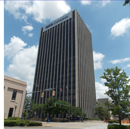
Daniel Building - 15 20th St S Purchaser: UAB 316,404 SF (vacant during 2023)
