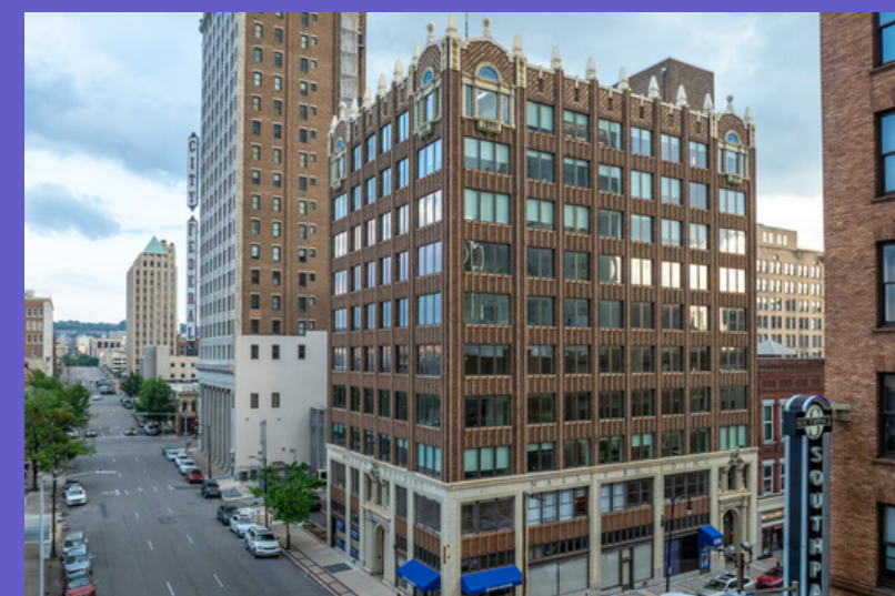
Massey Building - 2025 3rd Ave N Lessee: Singleton Schrieber 6,091 SF (signed September 2025)
