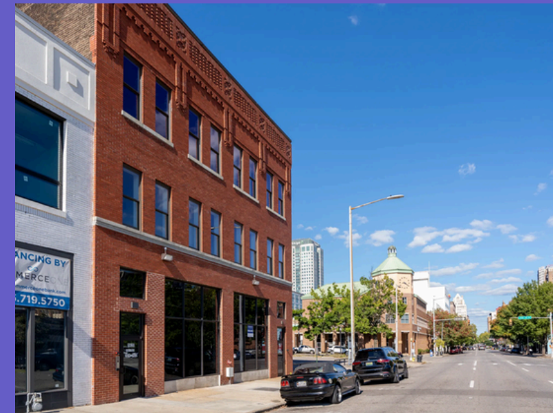
The Edison Building - 1620 3rd Ave N 6,000 SF of Contiguous Space Available
